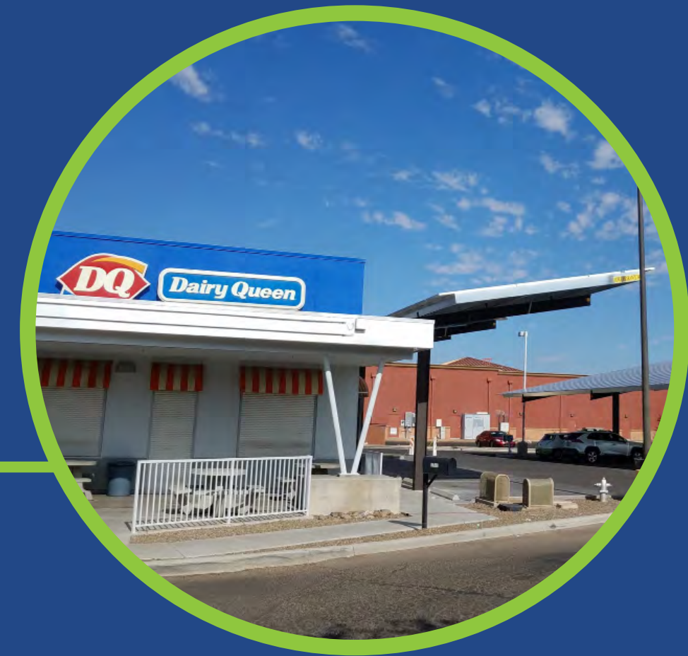
Dairy Queen System Size: 93 & 59 kW
